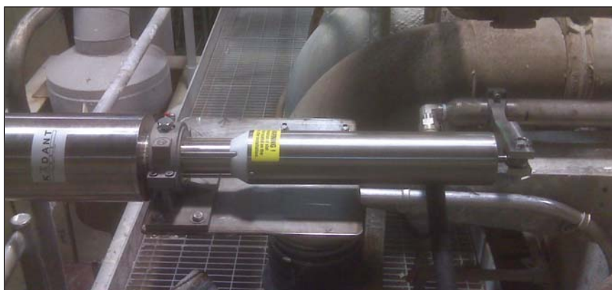
Genesis Oscillator Installation
