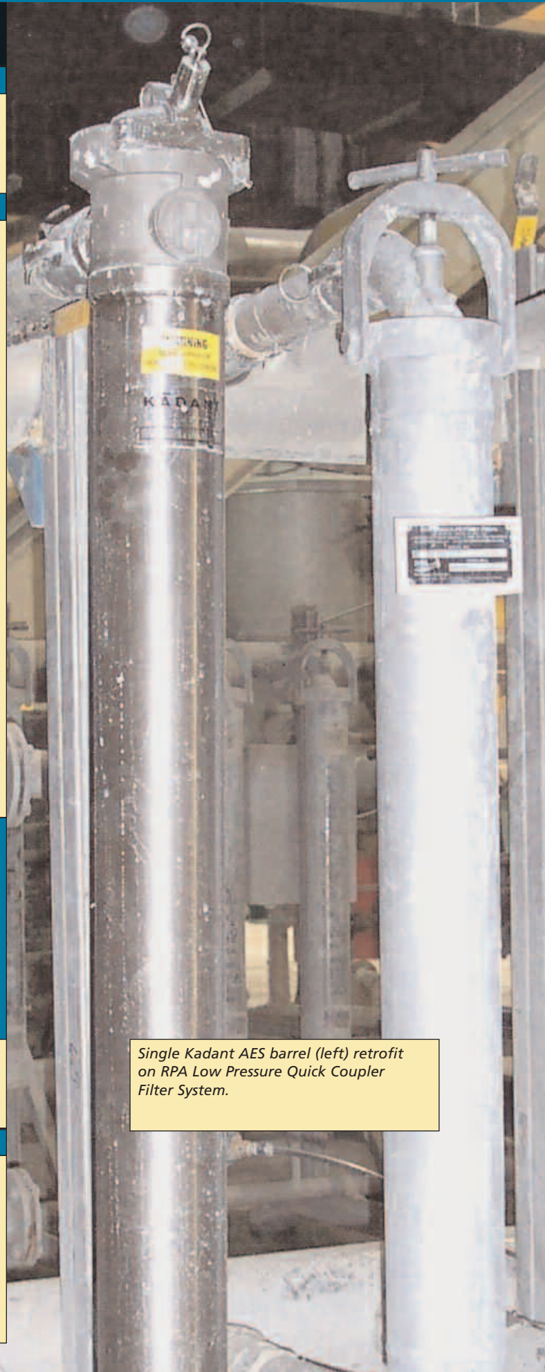
Kadant AES filter barrels with high pressure flanges (left) replace RPA barrels with quick couple connections (right).
